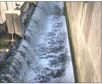
Activated carbon filtration was replenished with new media to enhance the extra layer of protection to remove any remaining contaminants after the biological process of treatment.
