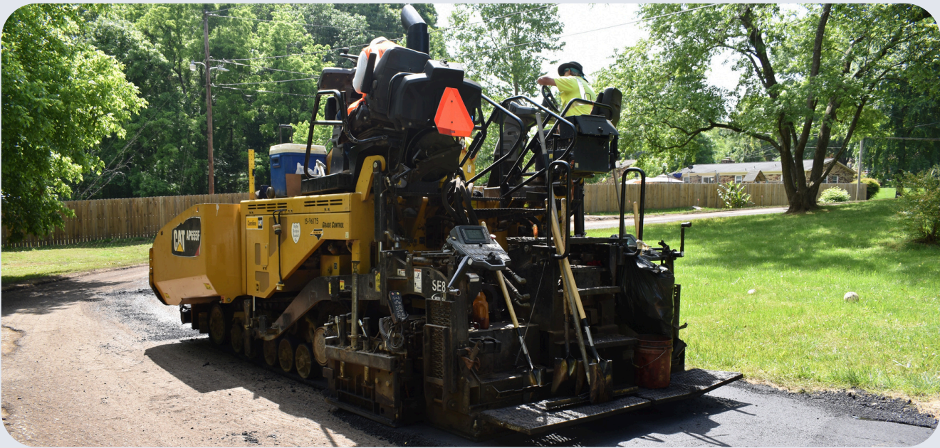
Pictured: Street resurfacing funded by 2022 GO Transportation Bonds
