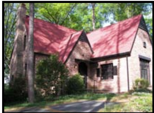
Retain Roof Shape
