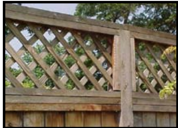
Wood Privacy Fence
