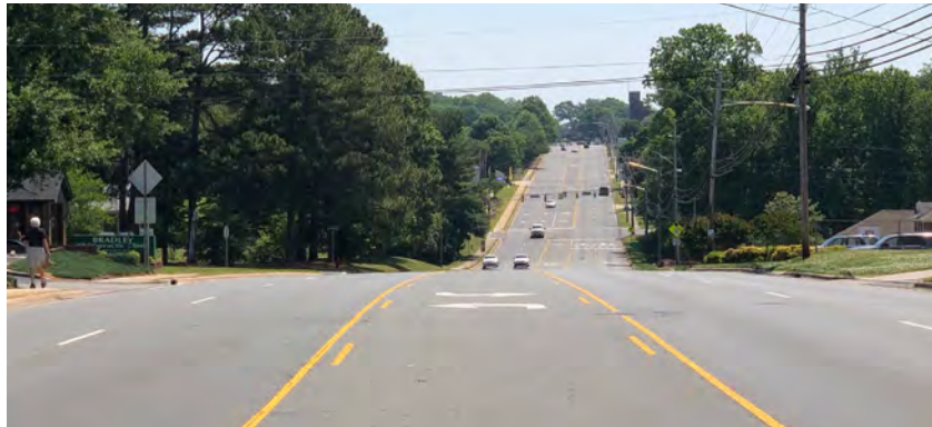
FIGURE 36: TYPICAL CONDITIONS ON GARRISON BOULEVARD
