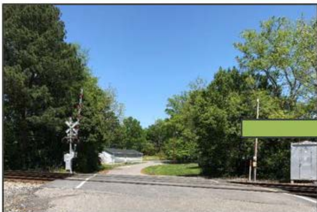
Figure 3: Skewed Railroad Crossing
